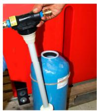
Taking the riser tube and distributor assembly, gently pull the rise tube out of the vessel head. There are 2 rubber "O"rings located within the female recess that accommodates the riser tube. Ensure on re-assembly that the riser tube is pushed gently but firmly home into the head assembly. This will ensure a water tight seal and prevent "tracking" of hard water to service flow.
